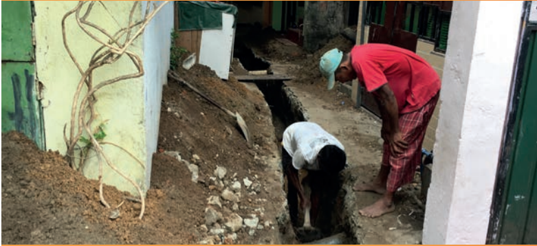
Construction of new main sewer line in 248 settlement, Sri Sangaraja Mawath, Colombo.
